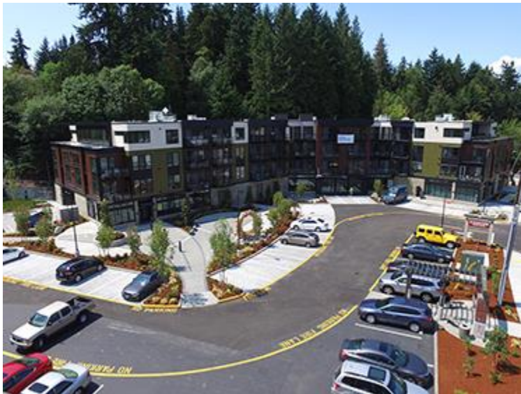
Photo provided by Henbart LLC enlarge
